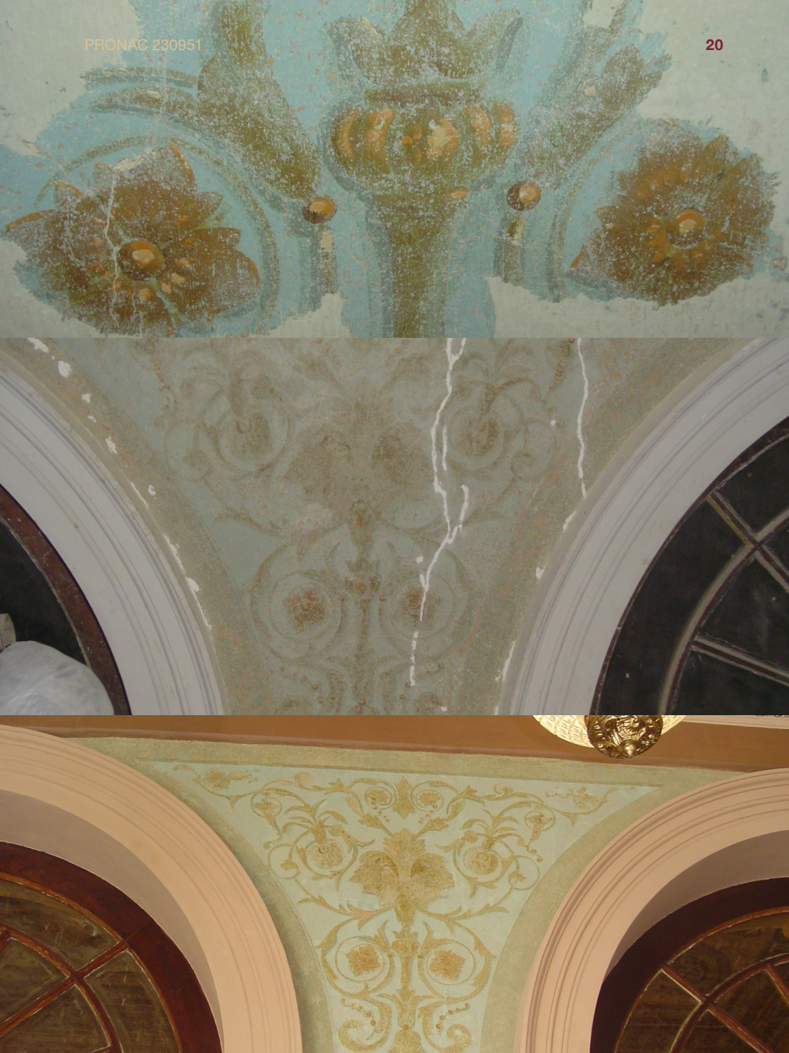
FIGURE 7 – Set of photographic records (before, during and after restoration), Rear Veranda painting LINK: Photographs for publication SOURCE: Personal archive of Tatiana Penna.
