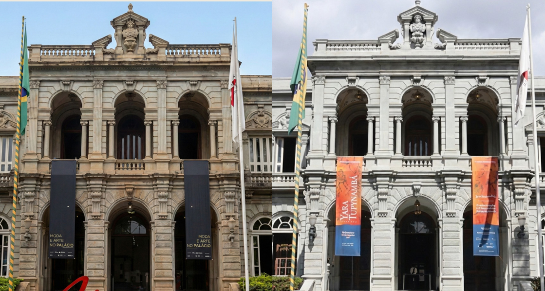
FIGURE 9 – Front Façade before and after restoration
